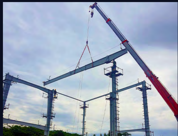
Proses Lifting Balok Baja Struktural
